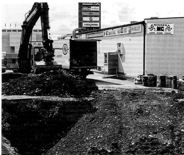
Figure 1.5 The soil under a gas station is removed as the site is remediated. Photo: Lars Ryden.
