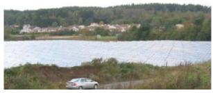
Figure 1. Solar panel field in Kungälv, Sweden - 10 000 m<sup>2</sup> delivers 4 million kWh heat per year to district heating
