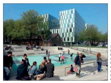
Figure 11.2 Dry detention pond. Benthemplein water square in Rotterdam, the Netherlands. Photo during dry weather. Can accommodate nearly 2 million litres of water during rain.
