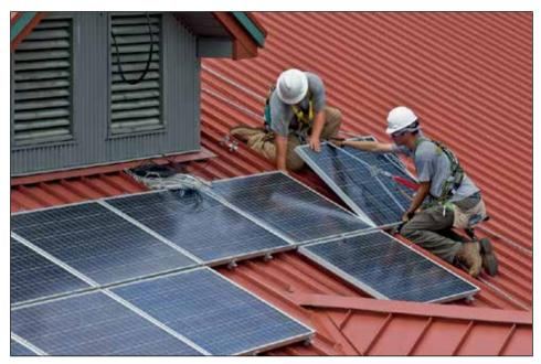
Figure 8.6 Installing solar cells. Source: Wayne National Forest Solar Panel Construction
