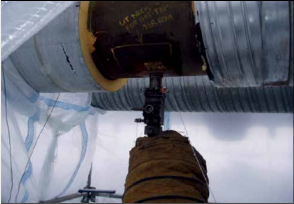
Figure 14.8. Insulation. Energy efficiency requires that pipelines are well-insulated. (Photo: Waska Williams Jr. – North Slope Borough)
