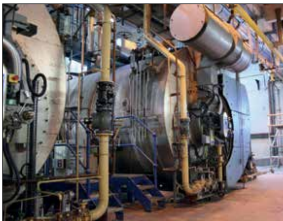
Figure 14.3 Boilers. Boilers, mostly for providing hot water, are basic in most energy systems. In smaller or medium sized industries, residential areas or large buildings, boilers in the size of 100-1,000 m 3 with output energy of 10-500 MW are common. The proper maintenance and use of boilers is important for energy efficiency. Further improvement is possible by using a cogeneration equipment in the scale proper – also small equipment are available – to produce both heat and power (electricity). (Photo: iStockphoto).
