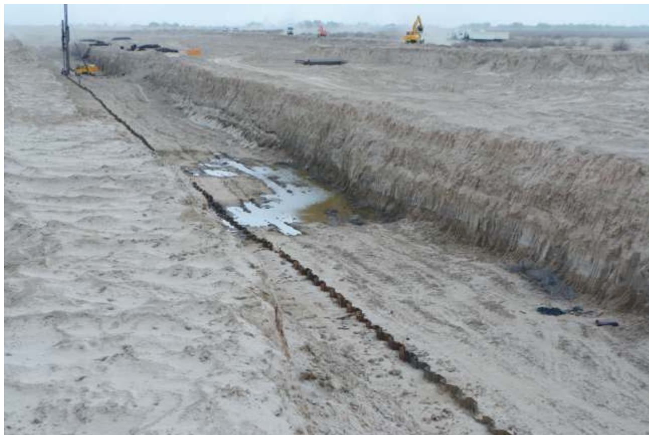
Spillway. Piling sheet pile into the base
