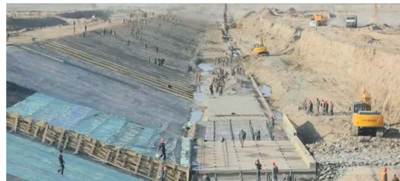
Construction of spillway structure from Maypost Lake to the Amudarya River
