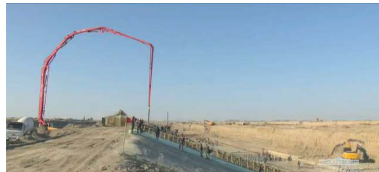
Construction of spillway structure from Maypost Lake to the Amudarya River
