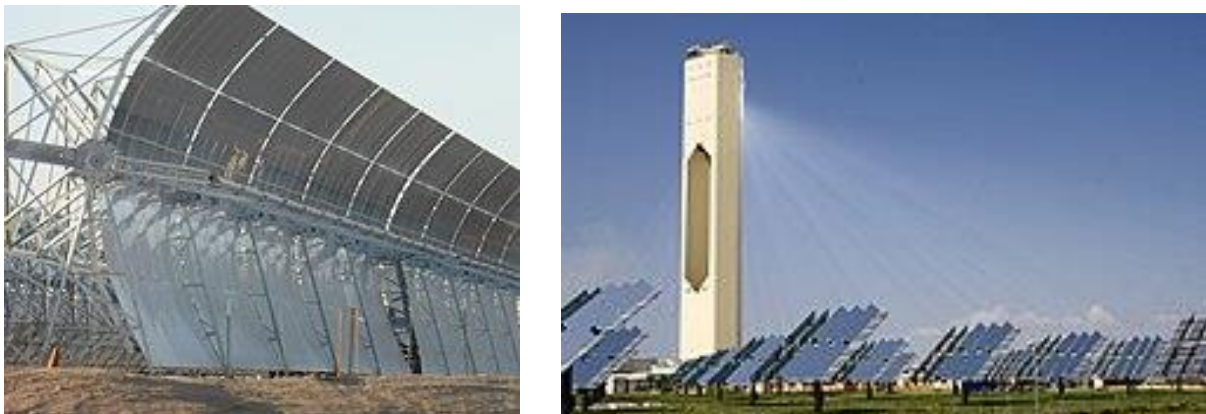
Figure 3. Left. Parabolic trough at a plant near Harper Lake, California ( https://en.wikipedia.org/wiki/Concentrated_solar_power#/media/File:Parabolic_trough_at_Harper_Lake_in_California.jpg )
