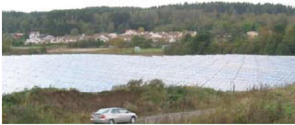
Figure 1. Solar panel field in Kungälv, Sweden - 10 000 m<sup>2</sup> delivers 4 million kWh heat per year to district heating
