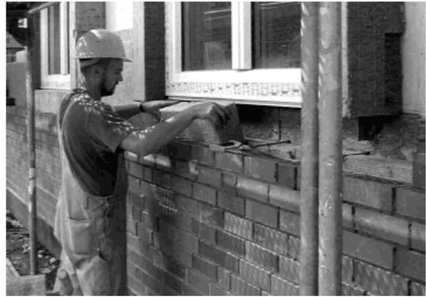
Figure 3. Passive house insulation with 20 cm core insulation.
