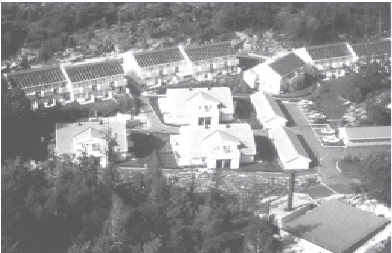
Figure 6.3 Solar collectors are especially suitable for central heating. The installation at Särö, south of Göteborg in Sweden, serves a small residential area of 48 apartments with 740 m 2 of roof integrated collectors in combination with 640 m 3 of water in an insulated steel tank placed in a rock pit. The installation, in operation since 1989, covers 35 % of annual load and 400 Mwh/y. It would cover 65 % if the storage was enlarged. (Source: Dalenbäck, J-O, 1996) (Photo Alpo Winberg).
