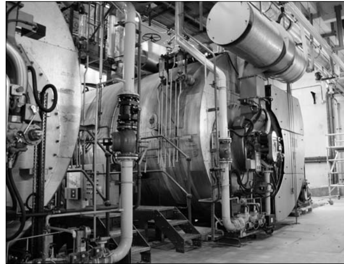
Figure 6.7 Boilers. Boilers, mostly for providing hot water, are basic in most energy systems. In smaller or medium sized industries, residential areas or large buildings, boilers in the size of 100-1000 m 3 with output energy of 10-500 MW are common. The proper maintenance and use of boilers is important for energy efficiency. Further improvement is possible by using a cogeneration equipment in the scale proper – also small equipments are available – to produce both heat and power (electricity). (Photo: iStockphoto)
