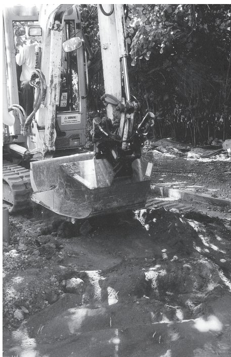
Figure 18.6. Removing soil. The most direct means for remediation of a contaminated site is to remove the contaminated soil and deposit it in a safe way. (Photo: Lars Rydén.)
