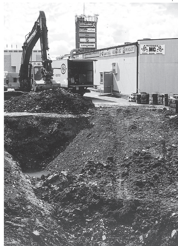
Figure 18.7. Old filling stations are sites where the soil is routinely monitored for chemicals before new uses. Here the soil under a previous gas station is being removed for a new residential house. (Photo: Lars Rydén.)
