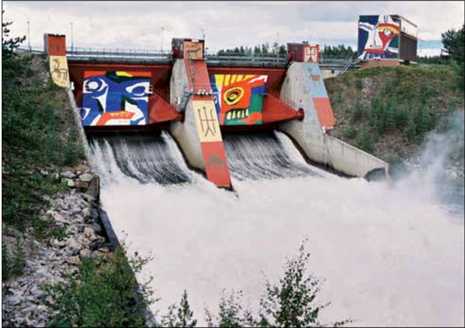
Figure 1.2 Hydropower. Akkats hydroelectric power plant in Swedish Lapland. Photo: Hans Blomberg
