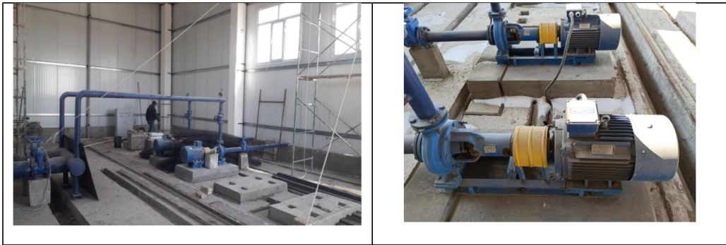
Pumping station building for installation of four pumps. In 2021 there were installed only two)
