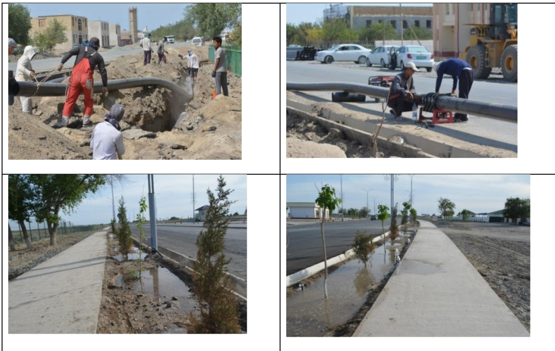
Construction of an irrigation pipe network in the city of Muynak
