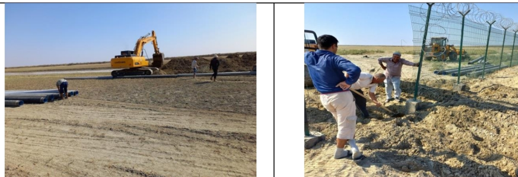
Construction of a closed horizontal drainage to protect the runway of Muynak airport from flooding from the Rybachy Bay
