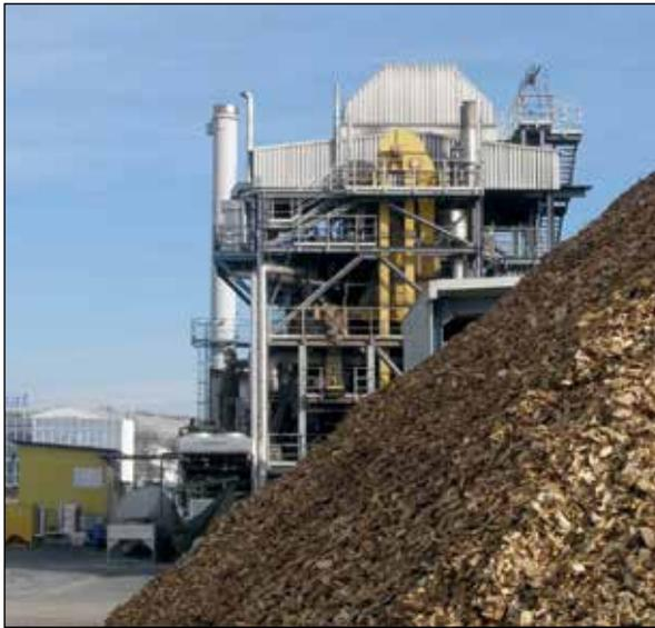
**Figure 12.2** Wood gasifier in commercial operation in Güssing. Photo: Gerfriede <https://commons.wikimedia.org/w/index.php?curid=1402990>
