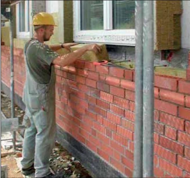
**Figure 8.5 Building a passive house.** The wall has extremely good insulation.
