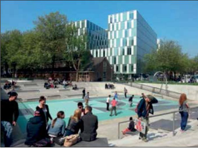
**Figure 11.2** Dry detention pond. Bentemplein water square in Rotterdam, the Netherlands. Photo during dry weather. Can accommodate nearly 2 million litres of water during rain.
