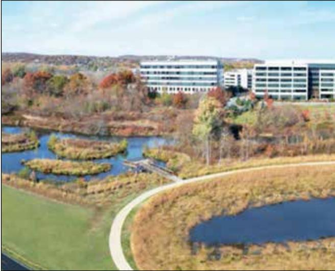
**Figure 11.4 Sedimentation – biofiltration system.** A large stormwater wetland in Massachusetts, USA
