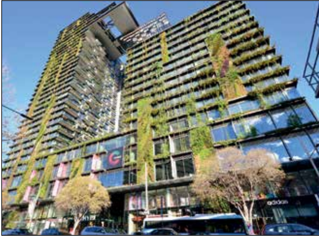
Figure 9.5 Green facades in Sydney Australia (Source: https://upload.wikimedia.org/wikipedia/commons/aa/%281%29Central_building_Broadway_Sydney-1.jpg )
