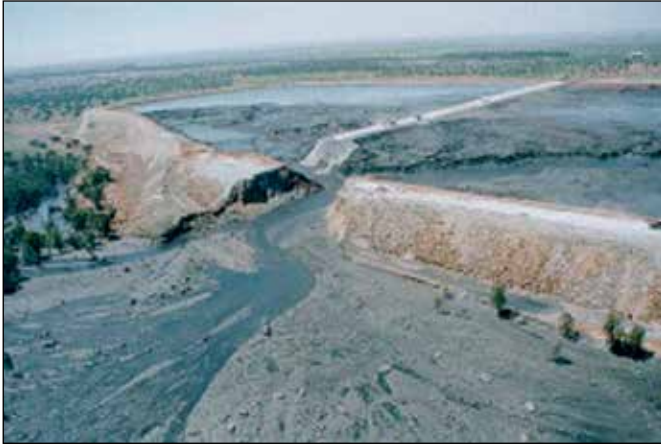
Figure 17.5 The serious pollution of the Danube River caused by a cyanide spill following a damburst of a tailings pond in Romania in 2000.
