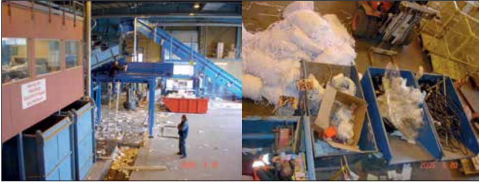
Figure 7.5 Semiautomatic paper sorting station (17 fractions)
