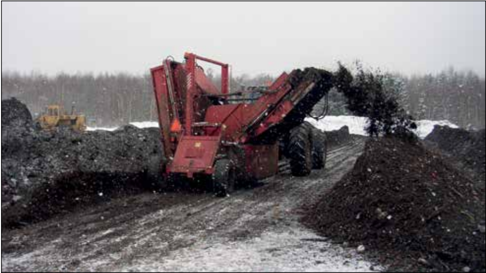
Figure 8.4 Processing of compost in the landfill in the town of Uppsala, Sweden
