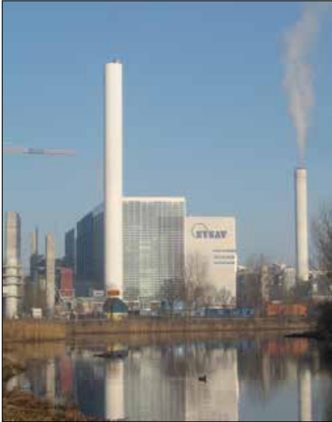
Figure 16.2 SYSAV incineration plant in Malmö, Sweden, capable of handling 25 metric tons per hour of household waste.
