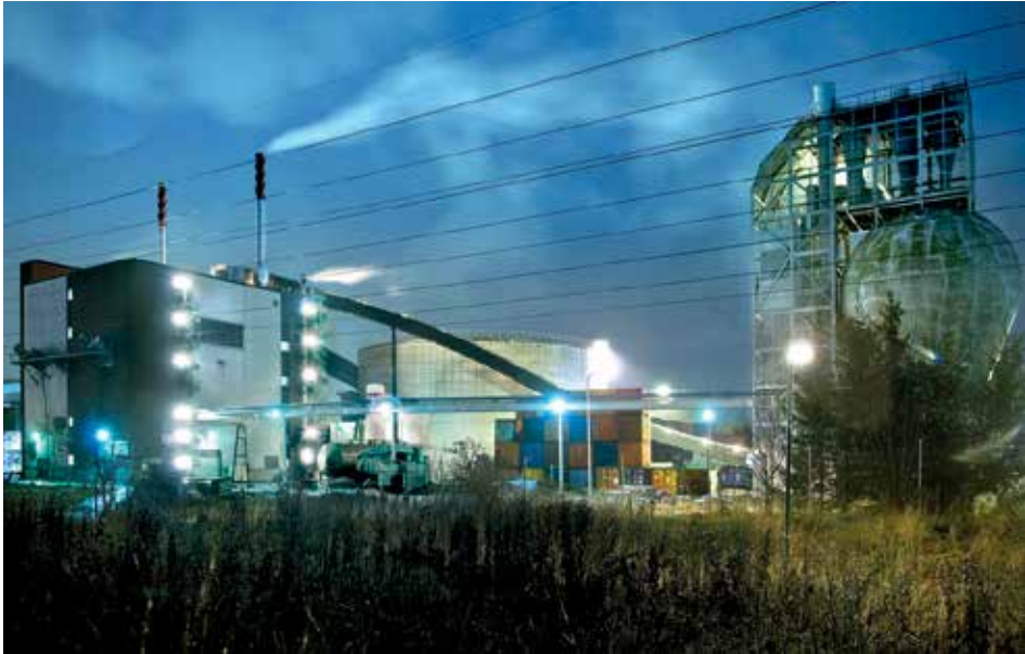
Figure 8.2 Incineration plant in Uppsala – one of many such plants operating in Sweden. This plant produces electricity and heat for the city and county with the population of about 500 thousand people. Environmental protection measures are the primary concern at the plant. Photo: Vattenfall.
