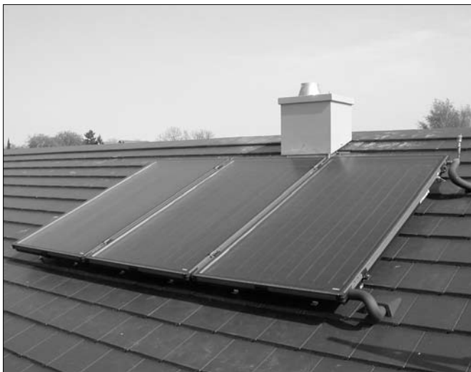
Figure 3.4 Solar panels. Warm water may be provided by using solar panels, a solution which is growing more economically competitive as the technology develops.
